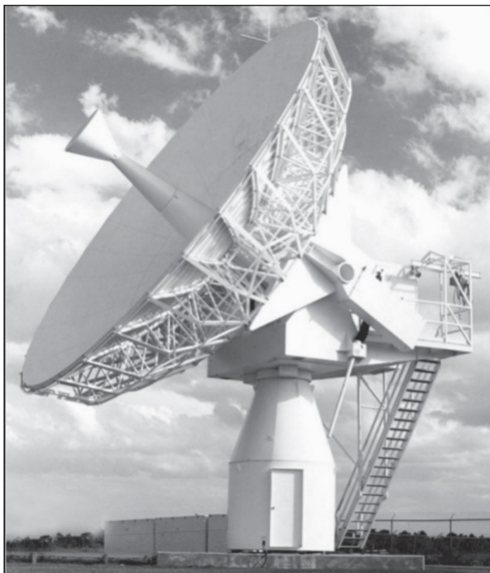
Figure A-5. AN/GSC-52(V) terminal
